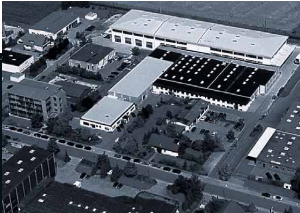
DORMA-Glas, Bad Salzuflen site. Situation in the '90s.
