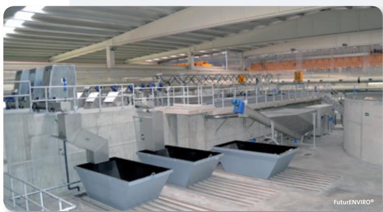
matter, and aid the settling of sand. Each blower is housed in a soundproof booth and controlled by a variable speed drive, in such a way as to enable a maximum airflow of 516 m<sup>3</sup>/h at a differential pressure of 4 wcm.
