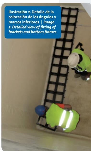
First of all, the arrangement of components was defined in accordance with the filter morphology and the position of the aeration ducts. The brackets were fixed to the walls to anchor the underdrain system and the bottom frames were fitted on top of the filter base.
