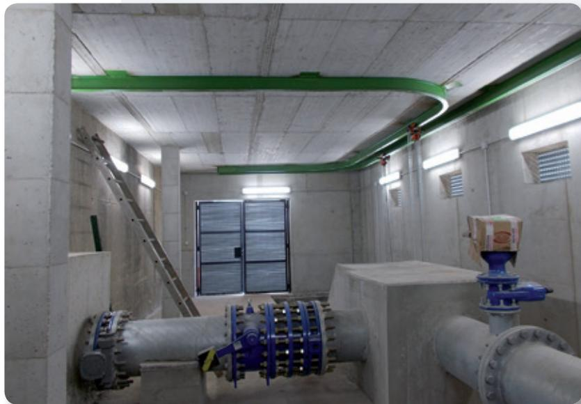
Owing to the quantity of pipes in the existing valve chamber and the difficulty associated with connecting the new pipeline with the two compartments of the tank, it was decided to build a new valve chamber on the northern side of the tank in order to effect the final connection between the pipeline and the tank. This chamber was fitted out with all handling and control elements necessary for correct operation.
