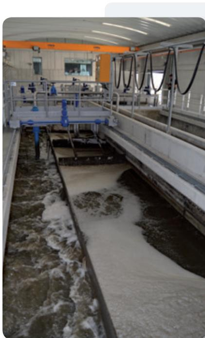
The grit extraction elements are arranged on the surface and consist of a vertical shaft centrifugal pump (1 per degritter) with a vortex impeller. Each pump is coupled to a mobile gantry crane and grit extraction is continuous along the length of the degritter.
