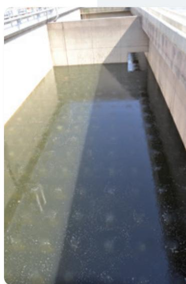
The anoxic zone, which is necessary for the denitrification of the nitrates generated in the oxic zone, is characterised by the absence of an external oxygen supply, with the only oxygen being that provided by the nitrates.
