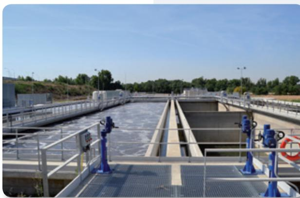
ensure that the plant effluent complies with established limits. The bioreactor comprises 2 identical, symmetrical lines, in which the compartmentalisation and the direction of the flow (U-shaped flow) ensure adequate plug flow.
