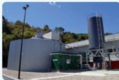
CAMBI SPAIN SLU, the Spanish subsidiary of CAMBI GROUP (Norway) supplied the Ourense WWTP with a thermal hydrolysis unit for pretreatment of sludge prior to anaerobic digestion.
