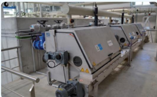
Aqseptence Group (formerly Bilfinger Water Technologies) supplied the Ourense WWTP with a number of units for sludge screening and subsequent drying from its brands Passavant and Noggerath ranges. 3 Noggerath RSH-E rotary drum screens featuring wedgewire 2.5mm screens, a screw conveyor and a waste compactor-cleaner were installed. The result is a reduction in sludge volume of up to 80% and an output dryness of 35-40%.
