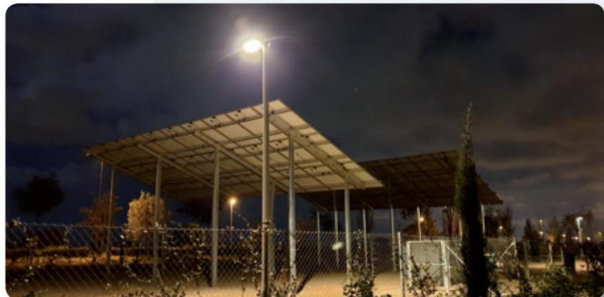
the decision was taken to power one third of these street lights via accumulation devices that are automatically programmed during the night by means of a solar clock.
