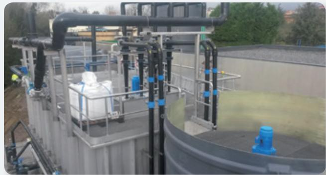
that were not treated due to lack of capacity at the WWTP. The solution adopted also meant that the works did not interfere in the operation of the existing plant. This is because one of the features of this technology is a small footprint, which enabled it to be installed in the limited space available on the grounds of the existing plant.
