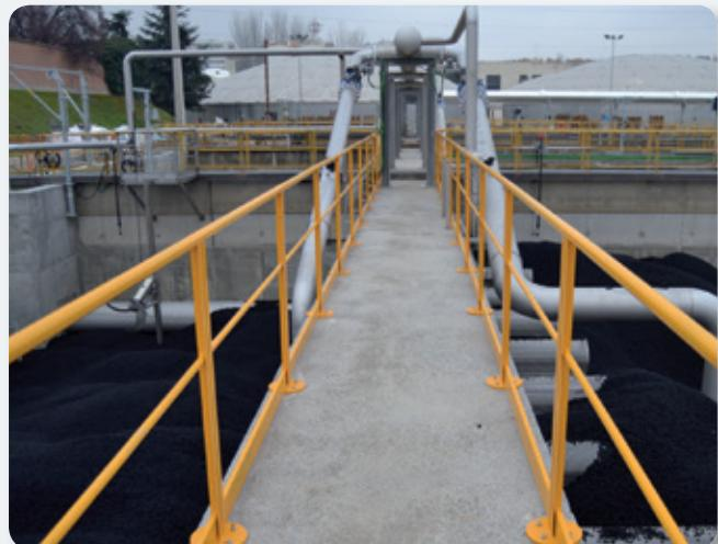
the subsequent assembly of the equipment necessary for the new process meant that the biological treatment line had to be stopped. The remodelling of biological treatment was carried out in two reactors at a time. Once the remodelling of the first two lines had been completed and the reactors put into operation, work began on the remaining two reactors.
