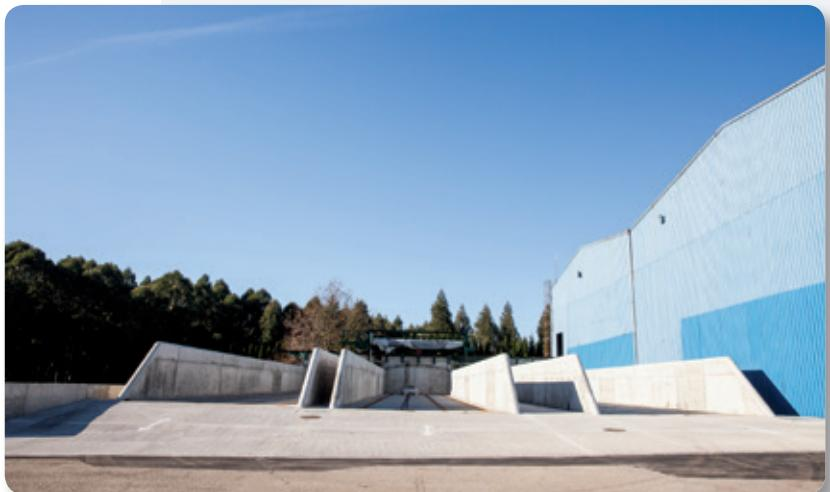
and irrigation systems to facilitate biological exchanges and the commencement of intensive fermentation. Parameters such as oxygen and temperature are automatically controlled within the trenches, thereby creating optimum conditions to accelerate the decomposition of the organic matter.
