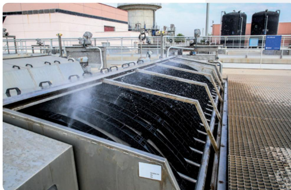
The clarified water is collected in a common channel, from where it is fed to the filtration lines. The filtration facilities are configured in two large lines that can operate independently. Each line treats a flow of 7,200 m<sup>3</sup>/h.
