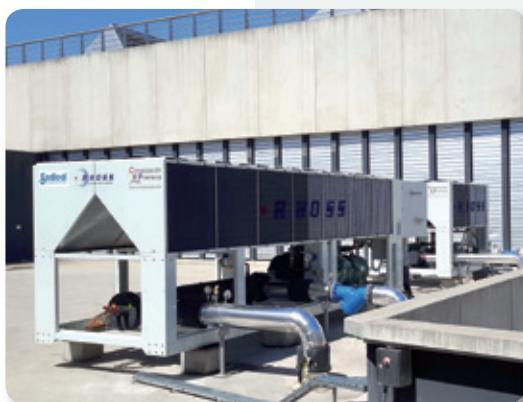
level of performance, controls the chillers. The integration of the chillers allows monitoring and action to be taken on key signals, optimising the operation and performance of the machines as well as taking full advantage of all the benefits of the CENTRAWebPlus system: internet connectivity and the option to send alarms via email.
