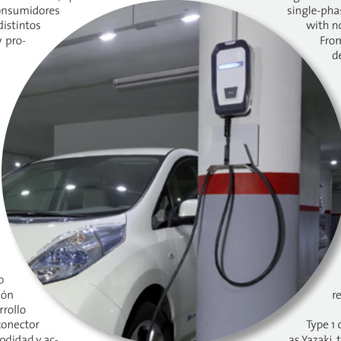
**Type 1 connector (SAE J1772):** also known as Yazaki, this is the Japanese standard for AC charging, also adopted by the US market and accepted in the EU. It has five terminals, three corresponding to the phase, neutral and earth with the last two as communication pins. One is a proximity sensor to prevent the car from moving while it is plugged in, and the other is for control and grid communication. It can work at up to 32 A in single-phase for slow charging.
