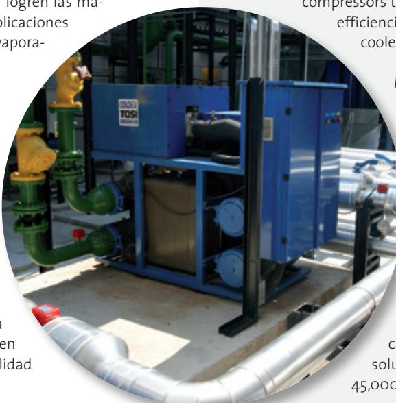
Magnetic bearings, two-stage centrifugal compression, a variable speed permanent magnet motor and intelligent electronic controls combine to create a sustainable energy efficient solution that is compact, lightweight and quiet.
