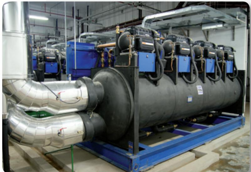
Turbocor® compressors are only half the size of a screw machine, thus reducing the space required for installation. The compressor's very low noise (72 dB) and zero vibration eliminate the need for insulation equipment. This reduces both the units' construction time and their installation costs. Moreover, the fact that Turbocor® compressors do not contain oil saves on after-sales maintenance.
