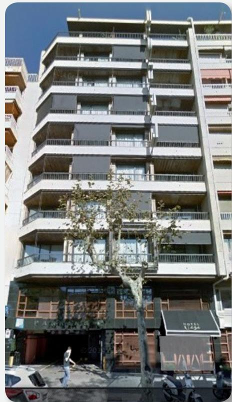
The installed solution comprised 35 motorised vertical black shades that absorb 96% of solar radiation while offering a high level of visual comfort as it is possible to see through the technical material thereby avoiding the cave or hideout effect of an enclosed space.
