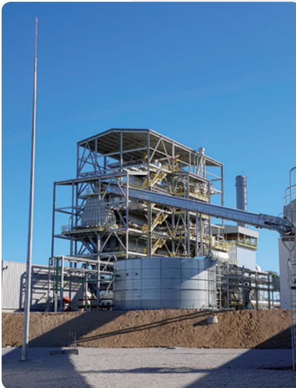
After the boiler and before the FDF, the gases are sent through a high-efficiency cyclone and bag filter prior to being released into the atmosphere. Finally, the gases are released at a temperature of less than 140°C through a double-walled stack. An AMS flue gas probe is installed in the shaft of the stack to continually measure gas emissions.
