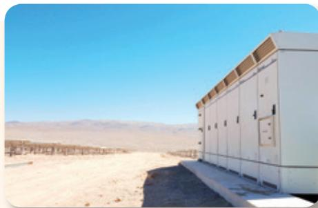
The HEC V1500 series includes the innovative iCOOL V cooling system that allows the inverter to work at up to 50°C at nominal power. The iCOOL V system smartly cools the inverter, regulating the cooling system capacity depending on the temperature sensors.
