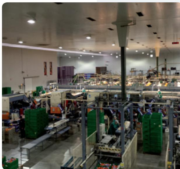
The existing floodlights and bell lamps in the main indoor working areas of the warehouse were HID 400W HAL type and have been entirely replaced by NEOS 3 LED 64L 99W NW, maintaining the necessary level of lighting at over 100 lux and increasing uniformity to 90%.
