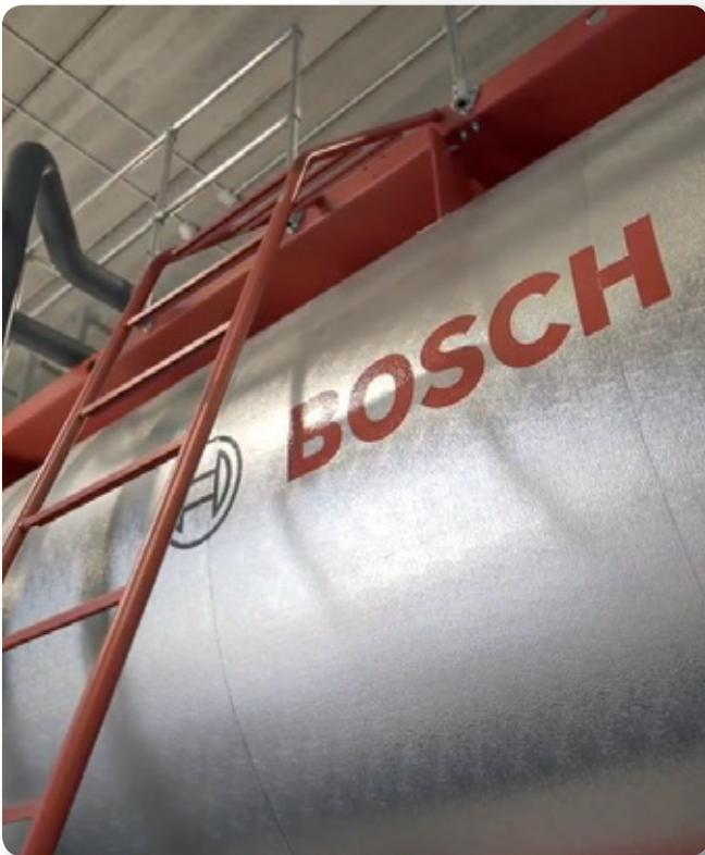
The three-pass smoke tube Unimat UT-L boiler is mainly used in hospitals, old peoples' homes, office buildings, residential complexes and in industry in general. Its high level of flexibility makes the UT-L ideally suited for use as a back-up boiler to cover peak loads in heating power stations and CHP plants.
