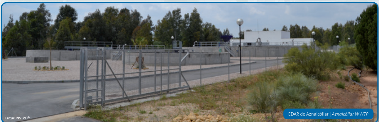
EDAR Guadalquivir | Guadalquivir WWTP
