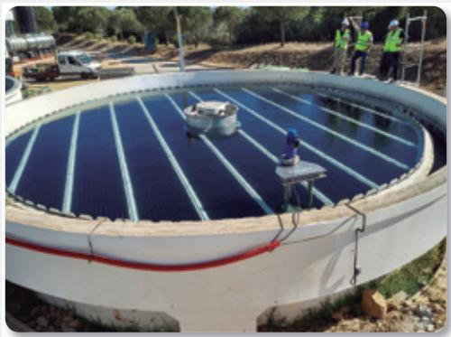
In order to increase the treatment capacity of the plant, TecnoConverting Engineering carried out all the clarification engineering involved in converting the 2 existing circular settling tanks and equipping them with TecnoTec H80 lamella modules. The result was an increase of 700 m<sup>3</sup>/h in the treatment capacity of the settling units.
