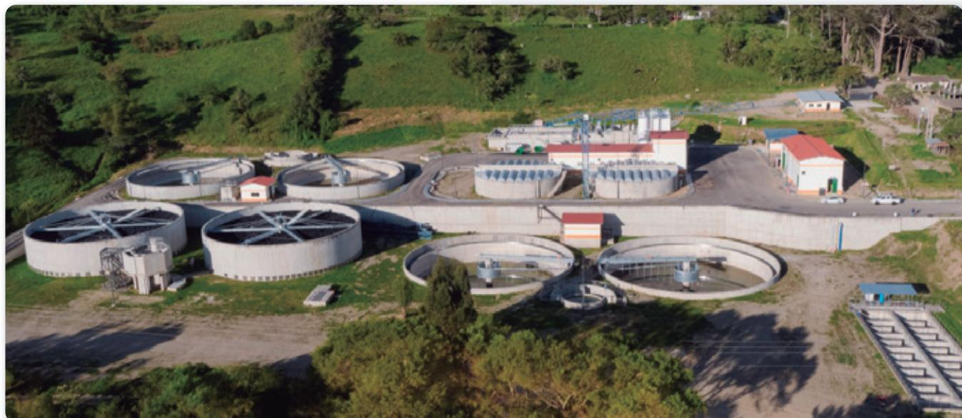
The trickling filter operates at an organic loading rate of 1.21 kg BOD5/m<sup>3</sup> per day and a hydraulic loading rate of 0.51 l/m<sup>3</sup>/s at the average flow rate. The filter medium has a total volume of 6,220 m<sup>3</sup>.
