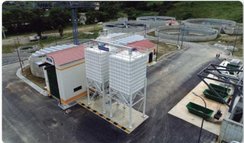
each is equipped with a 0.75 kW scraper bridge with peripheral traction.
